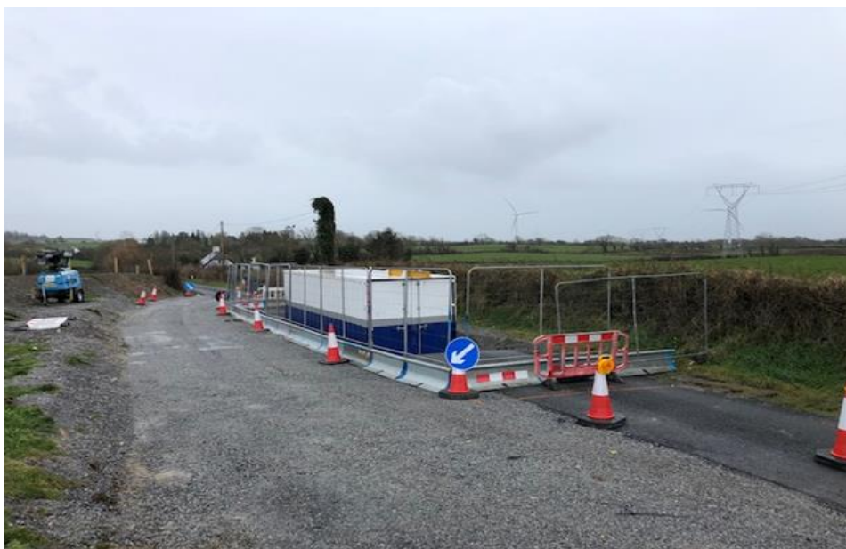
Figure 2.6: Typical HVDC Cable Jointing Bay Shelter
