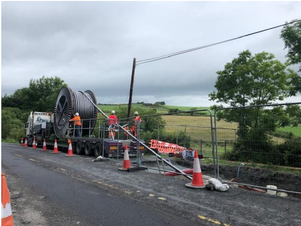
Figure 2.5: Typical Cable pulling at a joint bay
