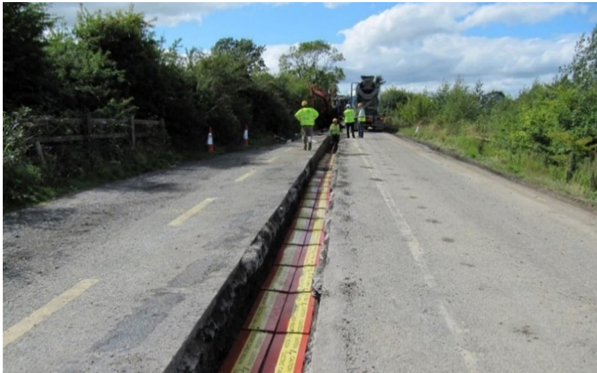
Figure 2.2: Typical HVDC Cable Trench in Road
