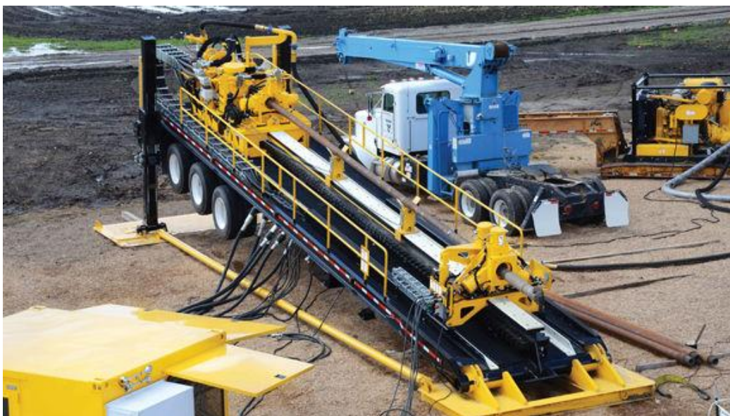
Figure 2.8: Typical HDD Drilling Rig
