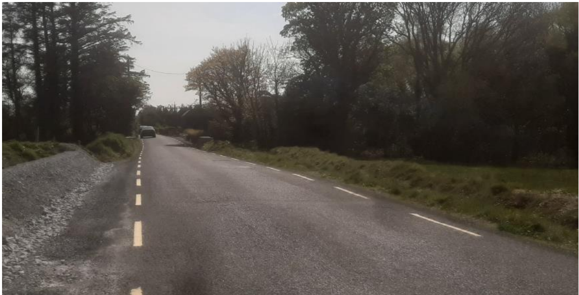
Figure 2.3: Reinstated road following laying of underground cables (UGC)
